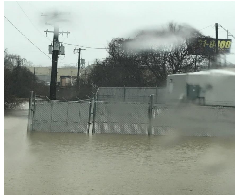
Chapman Highway Pump Station
