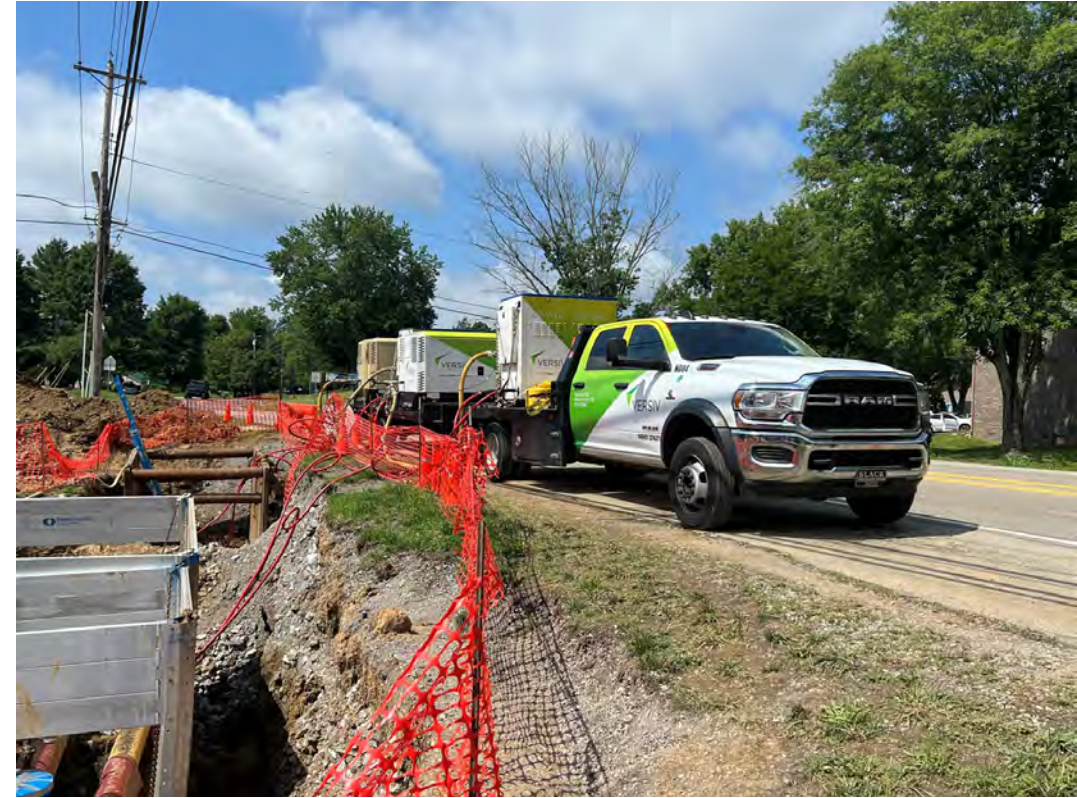
Cross-compression during Lovell Rd project commissioning
